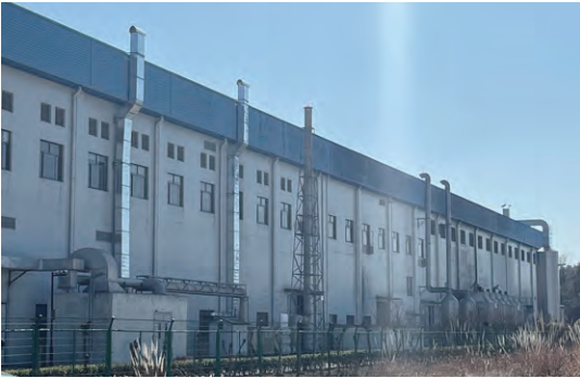
Exhaust treatment facilities of Li-ion battery factories
