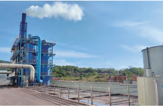
Exhaust treatment facilities of magnetic material furnaces
